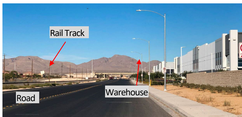
Figure 2: A warehouse with a rail track across a street [10]
